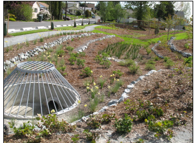
4th Ave S and S Trenton St. Storm Drainage Improvements, Seattle Public Utilities
